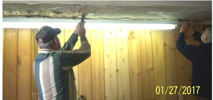
Carpets were soaked and ruined and had to be removed. The cellutex walls were saturated and had to be taken down to the original boards. Likewise several walls had to be stripped and inspected. The clubhouse is now in the "drying" stage and a committee is putting together a plan of action for renovation.
