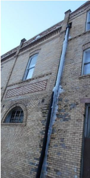
Leakage found its way into three floors. The first rupture occurred in the ceiling of the museum. Fortunately it occurred in an area of open space and did not cause damage to any exhibits. There will need to be sheet rock repair when we are sure there is no more danger of flooding.
